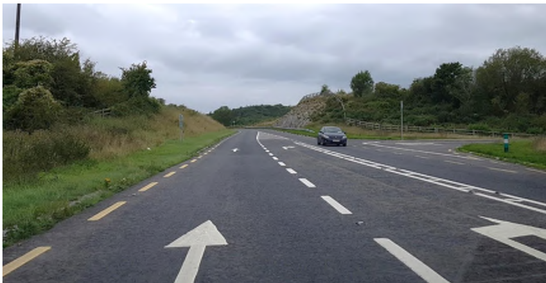
Plate 2.29 N69 west of Kildimo: Recent minor improvement scheme
