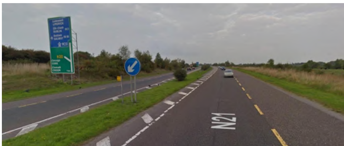
Plate 2.17 N21 Dual Carriageway Terminal – Change in Cross-Section (Source: Google Street View)
