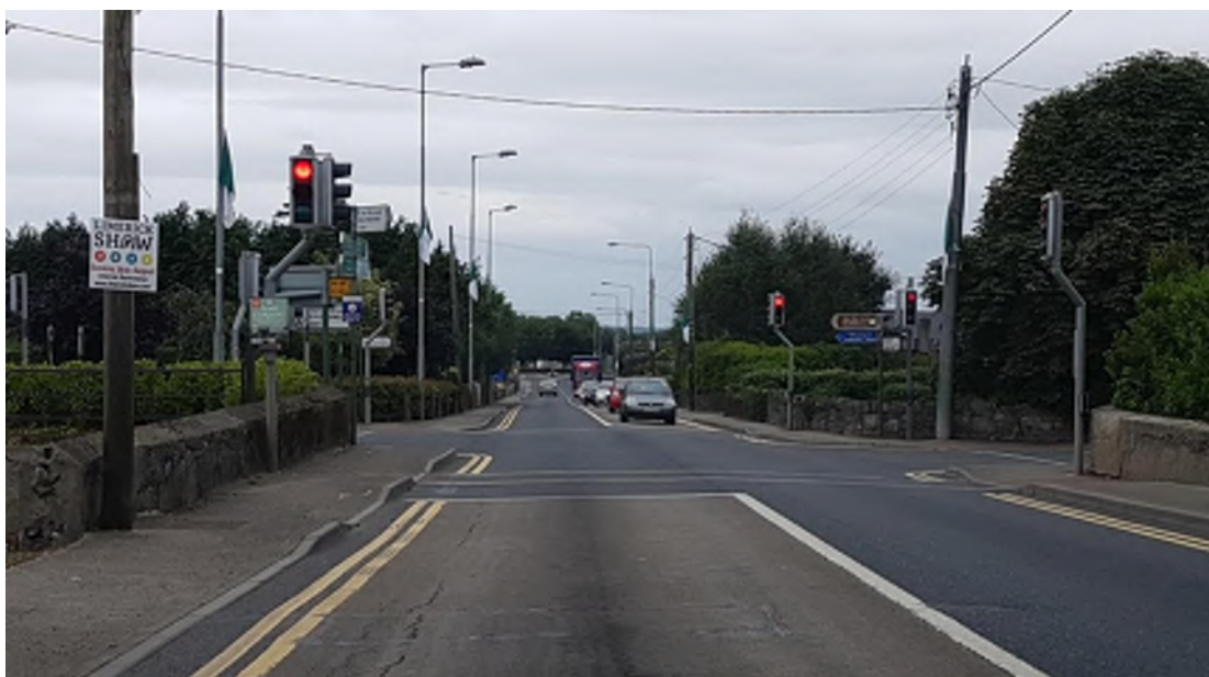
Plate 2.32 Traffic Signal on N69 in the village of Clarina
