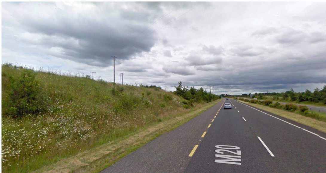
Figure 5.23 M20 Northbound carriageway between Junction 4 and Junction 3
