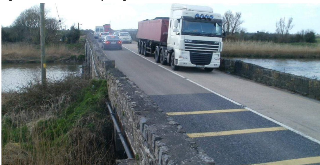
Figure 5.3 N69 at Ferrybridge
