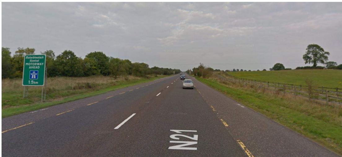
Figure 5.19 N21 between Lantern Lodge and Attyflin – Single Carriageway
