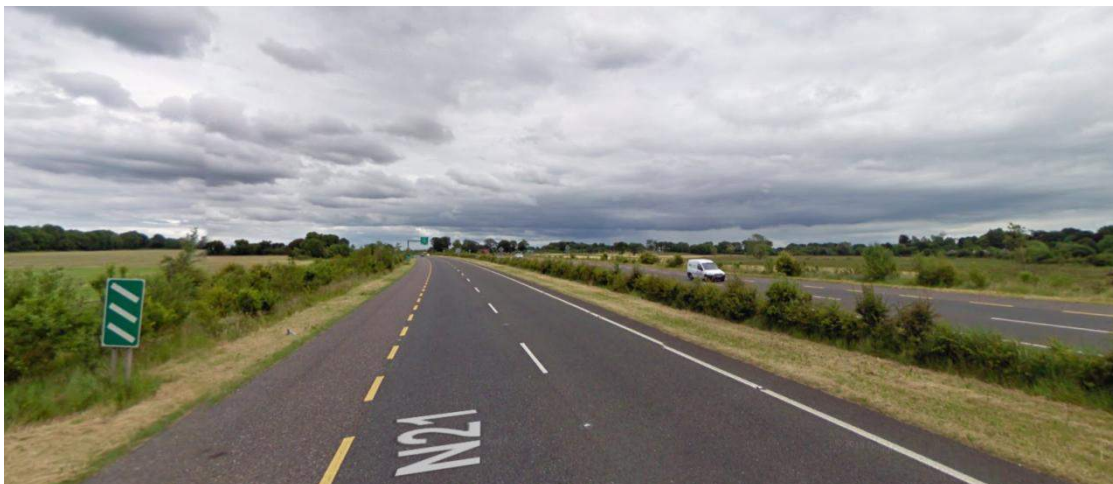
Figure 5.21 N21 between Lantern Lodge and Attyflin – Dual Carriageway
