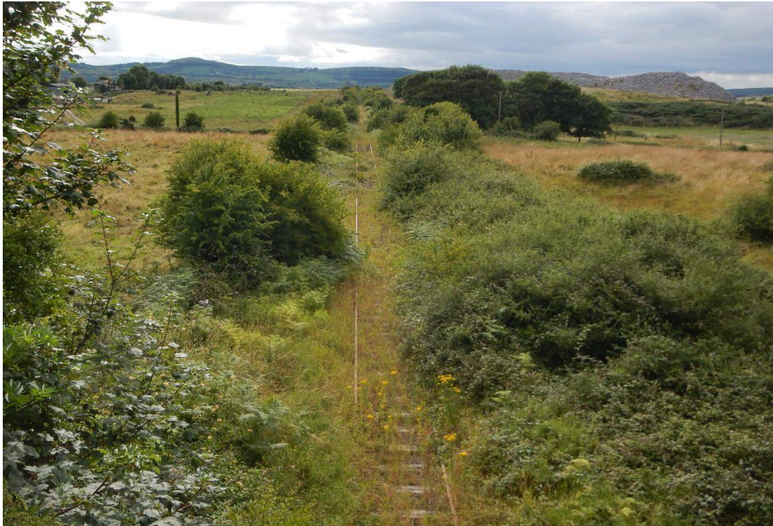
Figure 3.2 Foynes to Limerick Railway Line
